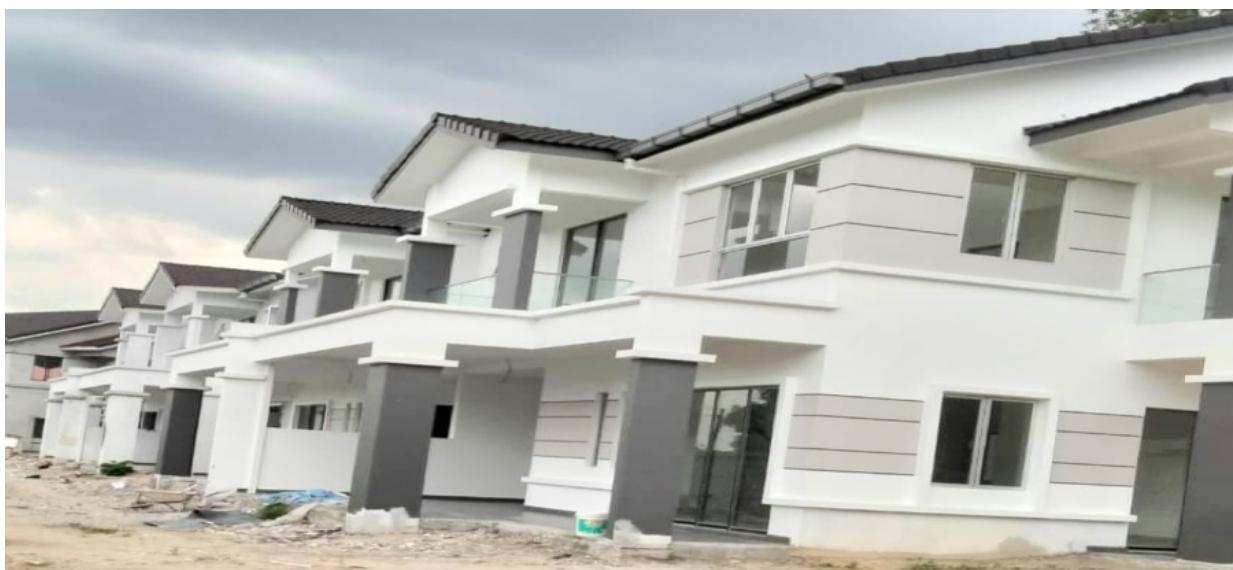
2-Storey Terrace Houses, Saujana Impian, Kajang, Selangor. (Construction works in progress)
