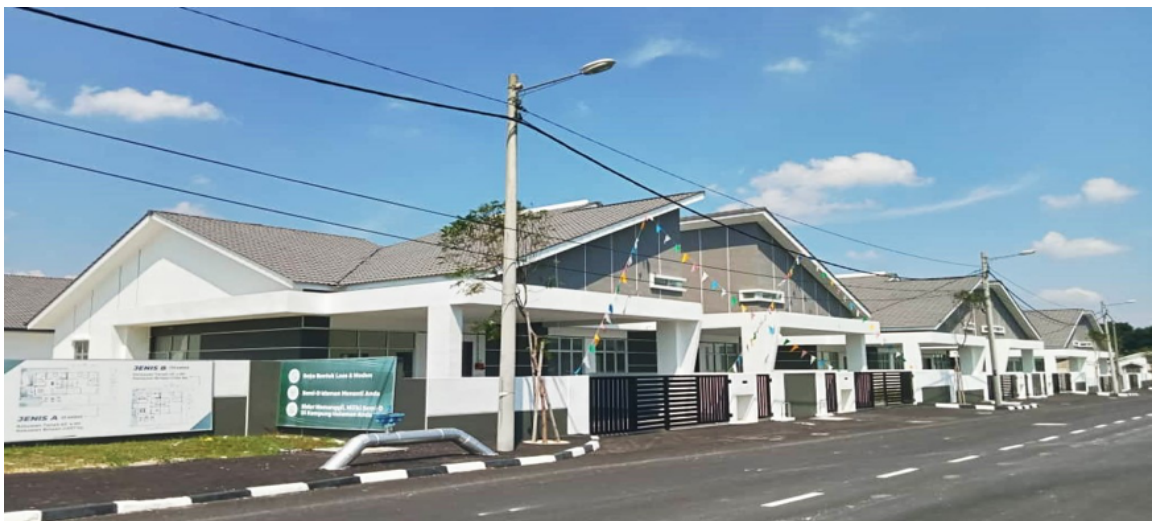
Phase 7A, 1-Storey Semi-Detached Houses, Taman Impiana Bidor, Perak. (CCC issued on 12 August 2025).
